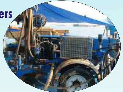
Bentonite Slurry Application
